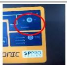
Turn OFF the DC ISOLATOR on the UNDERSIDE of each inverter (one for each inverter installed)
